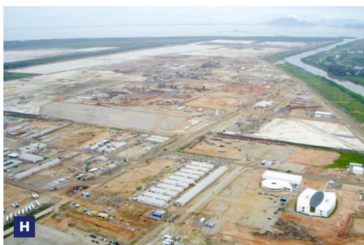
G Vista aérea da reclamation site of steel plant
